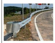
Guardrails are typically formed from slitted steel coils. They are used in construction of a boundary as a means to prevent or deter access from one side of the road or bridge to another.
